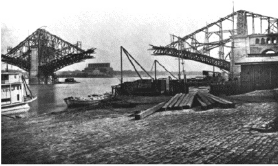
Eads Bridge under construction St. Louis, MO
